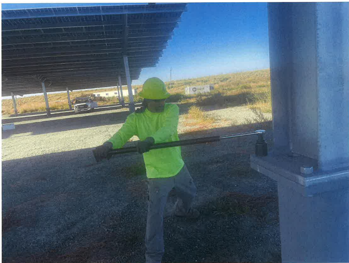
1110-0950: Twitchell Solar Project - Structural Steel Bolting
