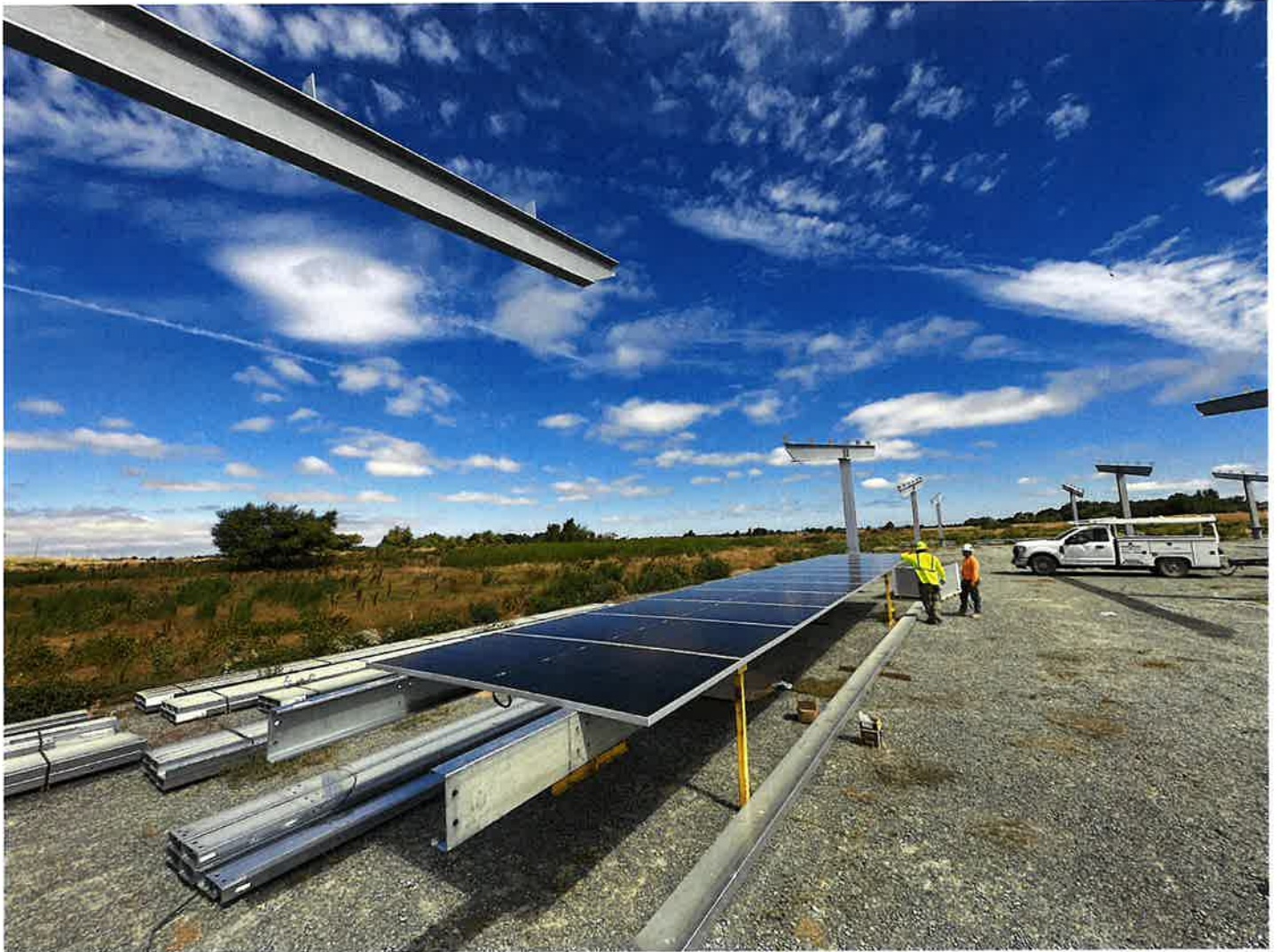
1110-0950: Twitchell Solar Project - PV Module installation
