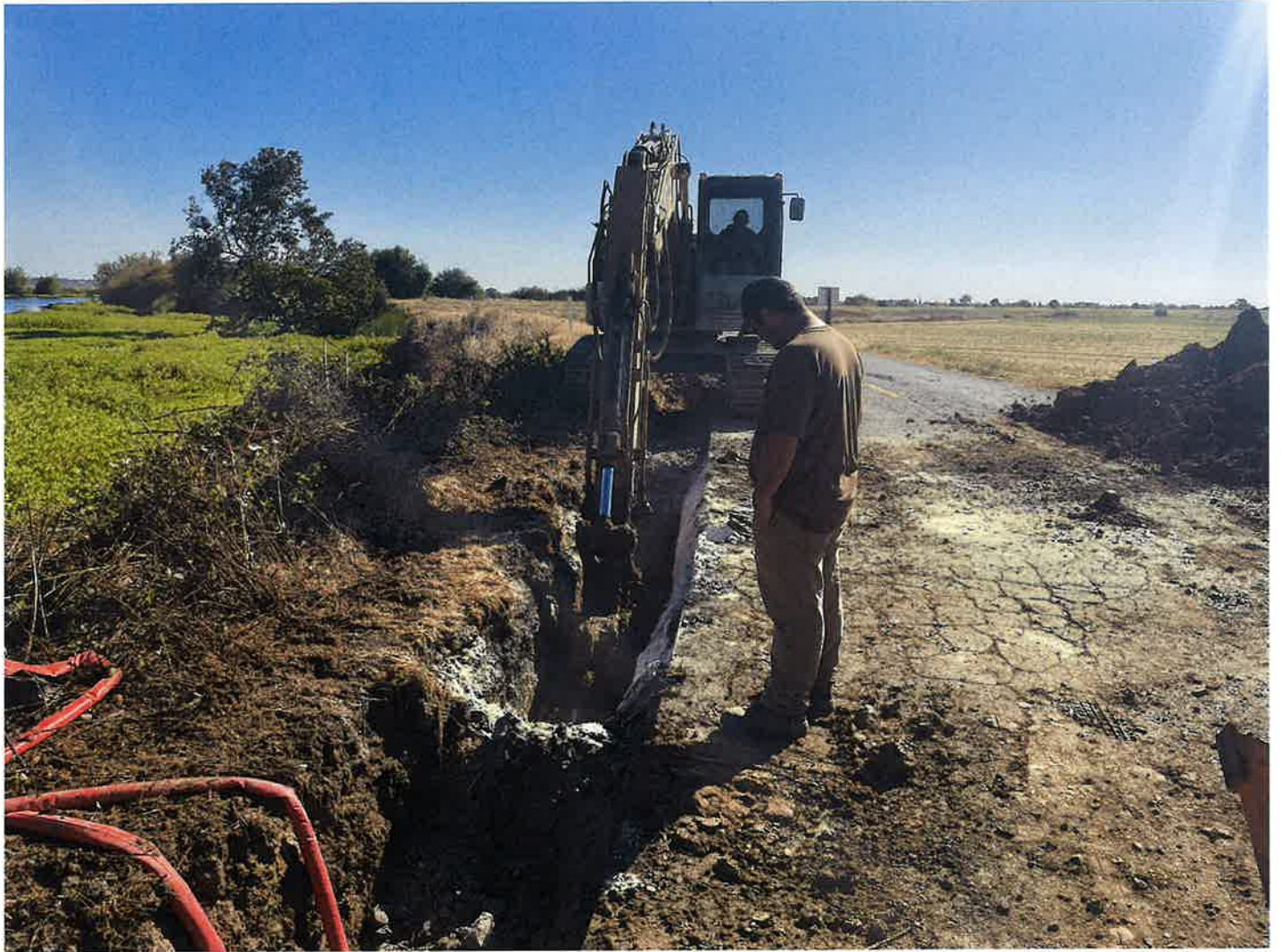
1110-9026: Station 236+00 Core Wall - Construction
