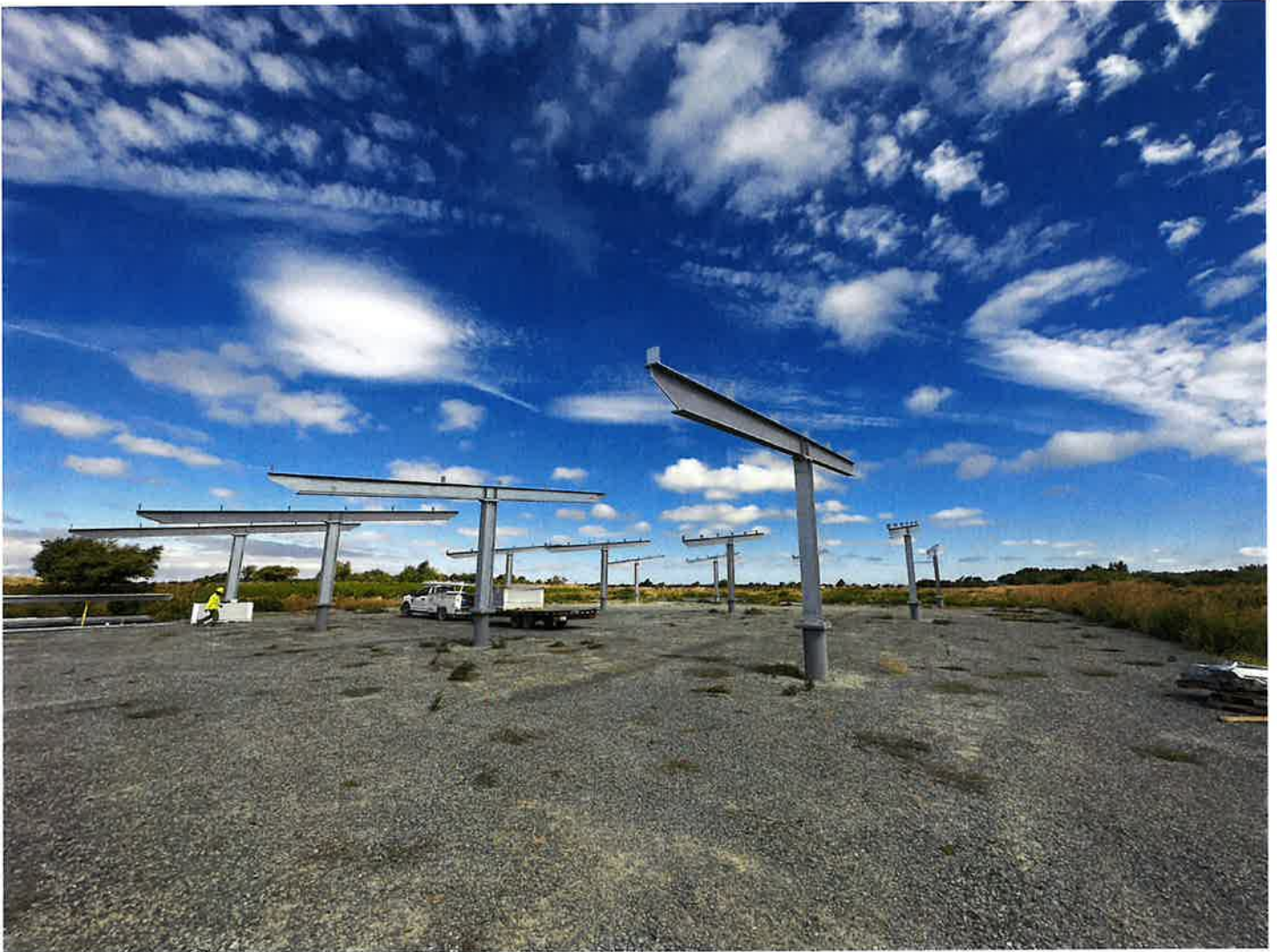
1110-0950: Twitchell Solar Project - Structural Steel Installation
